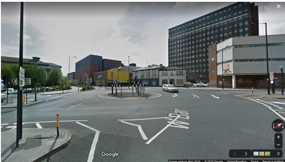
West Bar roundabout (7 accidents)
